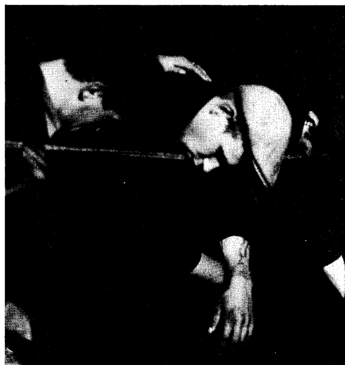
These men have paid to sleep 'on the line' in a warm room during the winter of 1930. The rope holds them up while they sleep.
